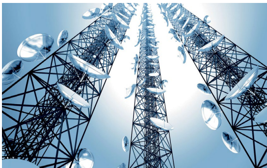
Telecommunication power supplies
